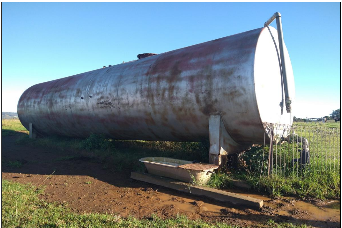
Photograph 8 - Former fuel storage tank reutilised for water pumping and storage. for farm animals (MRP132)
