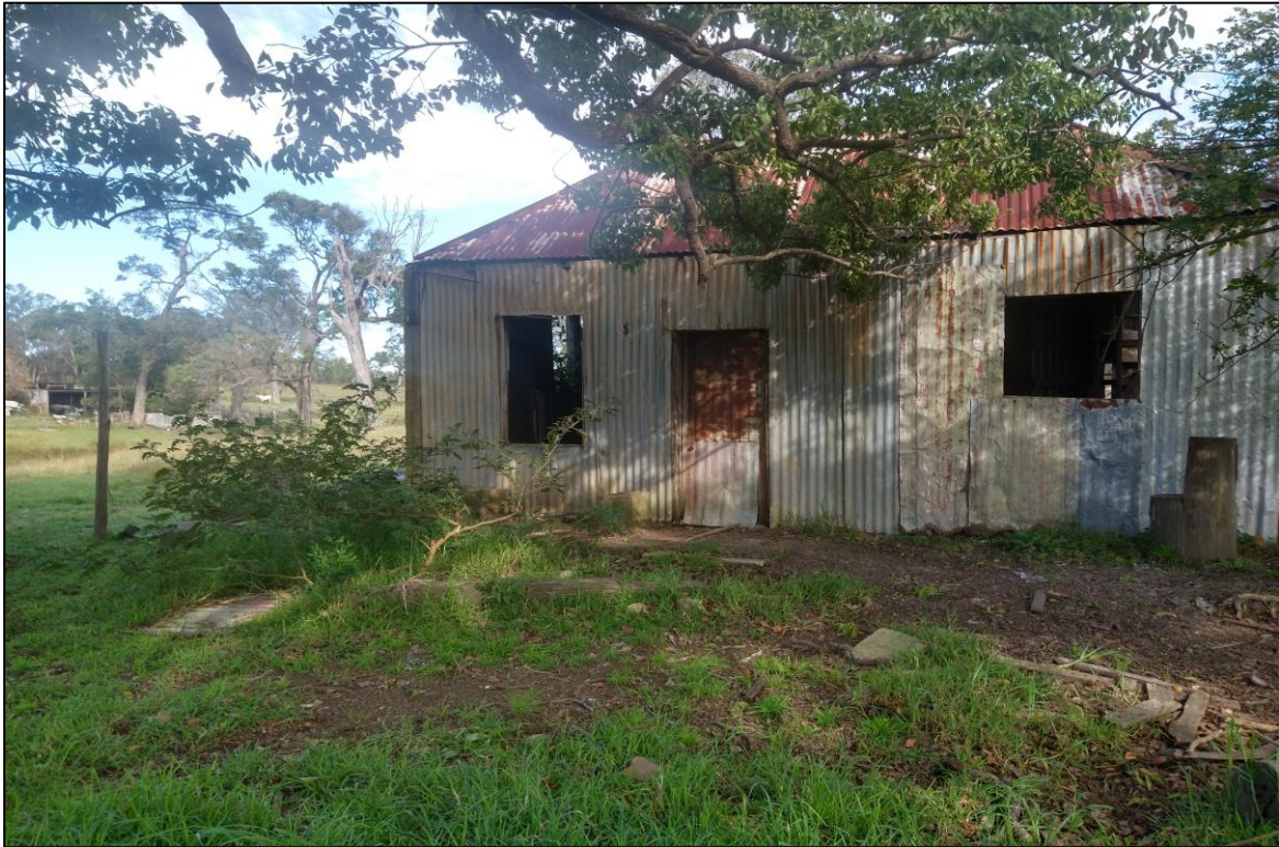
Photograph 29 - Dilapidated shed constructed of metal corrugated sheeting on an unsealed soil base observed in Lot 3, DP804375 (MRP 146).
